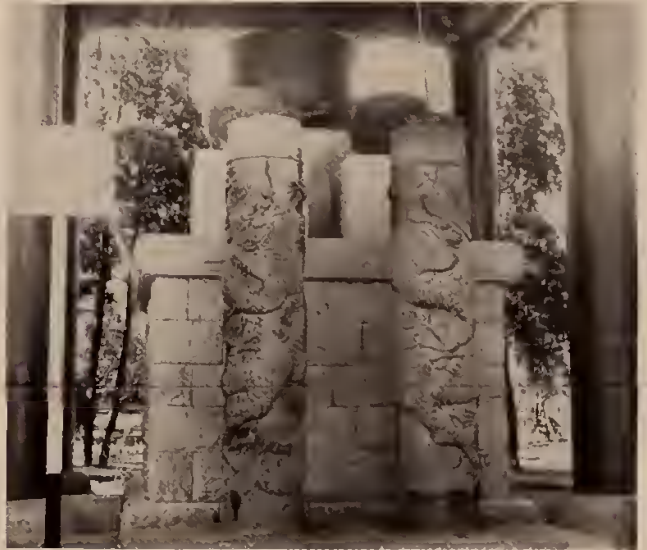
Water clock , supposedly one of two in existence, is at Seoul. Water trickles slowly from large vessel into smaller ones below it, thus raising a float which moves a marker which tells the time. Korean hour was 120 minutes, dividing their day into 12 hours.
